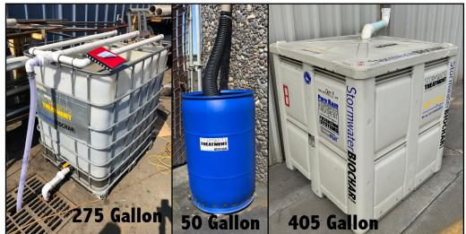
Transportation Company / Roadway & RR Runoff / Passive Box **Pure Rain**<sup>™</sup> Filtration System | Flow Type *Passive*
